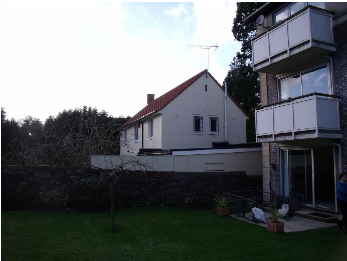
Existing property shown in relationship to closest flats of Severnleigh Gardens.
